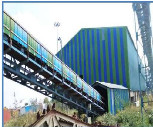
Gypsum storage shed & Closed conveying system
