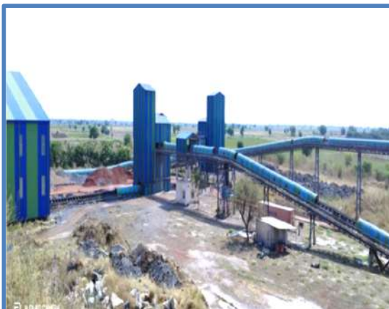
Closed limestone conveying system circuit
