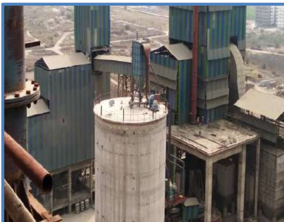
Bag Filters at Flyash silo Top
