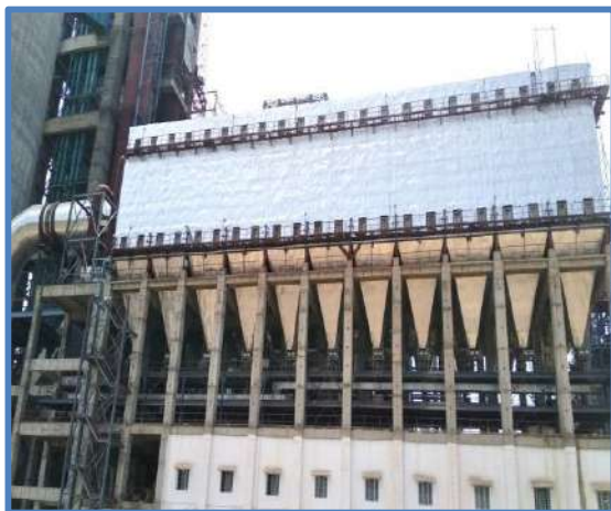
RABH for Kiln & Raw Mill
