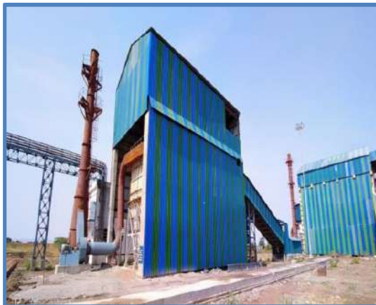
Bag Filter at L/S secondary crusher
