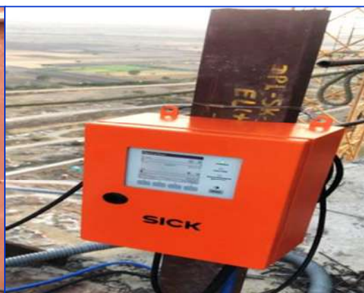
PM CEMS for Coal Mill Bag House Stack
