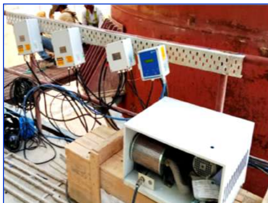
PM &amp; Gaseous CEMS for Kiln &amp; Raw Mill RABH Stack
